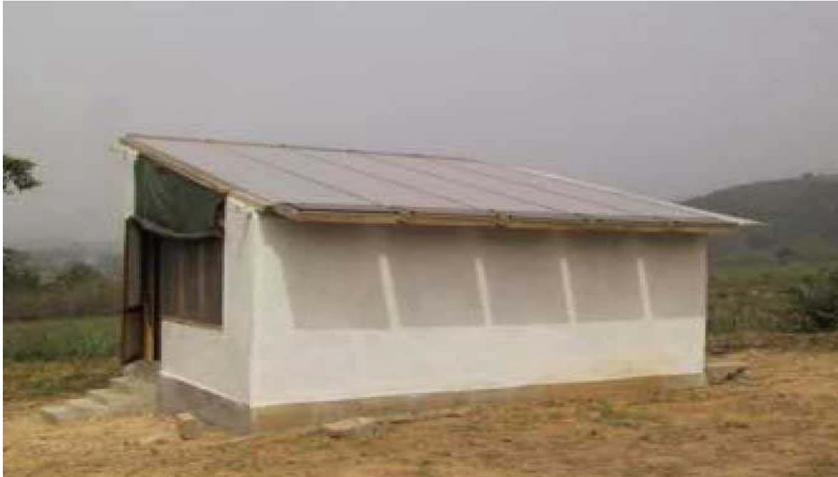
Fig. 35: In-house type solar crop dryer in Ghana [25]
